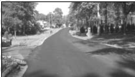
ARTS Project in Greenville County, SC West Golden Strip, Mauldin, SC
