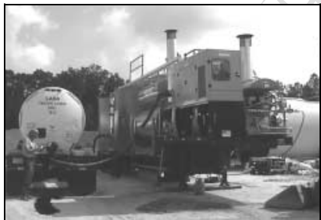
Pumping plain liquid asphalt into the blending unit.
